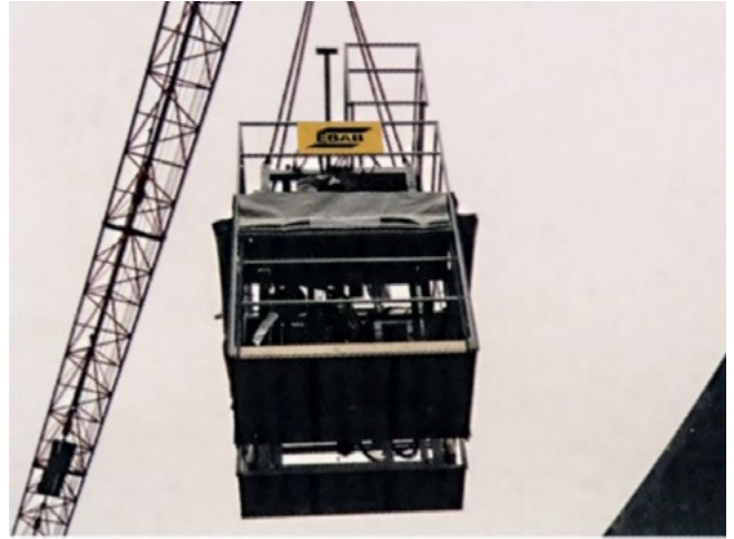
Double-side Circotech being lifted onto the job
